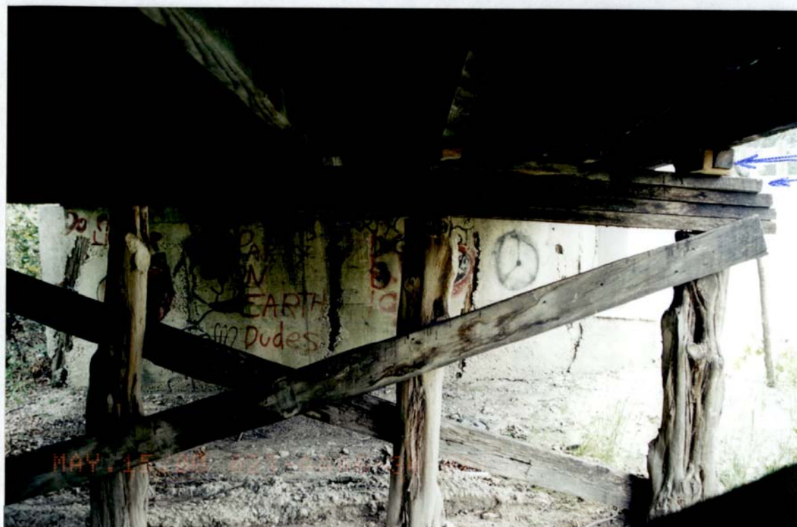
SOUTHWEST INTERIOR BENT - LOOKING SOUTHWEST (shoring Bent)
