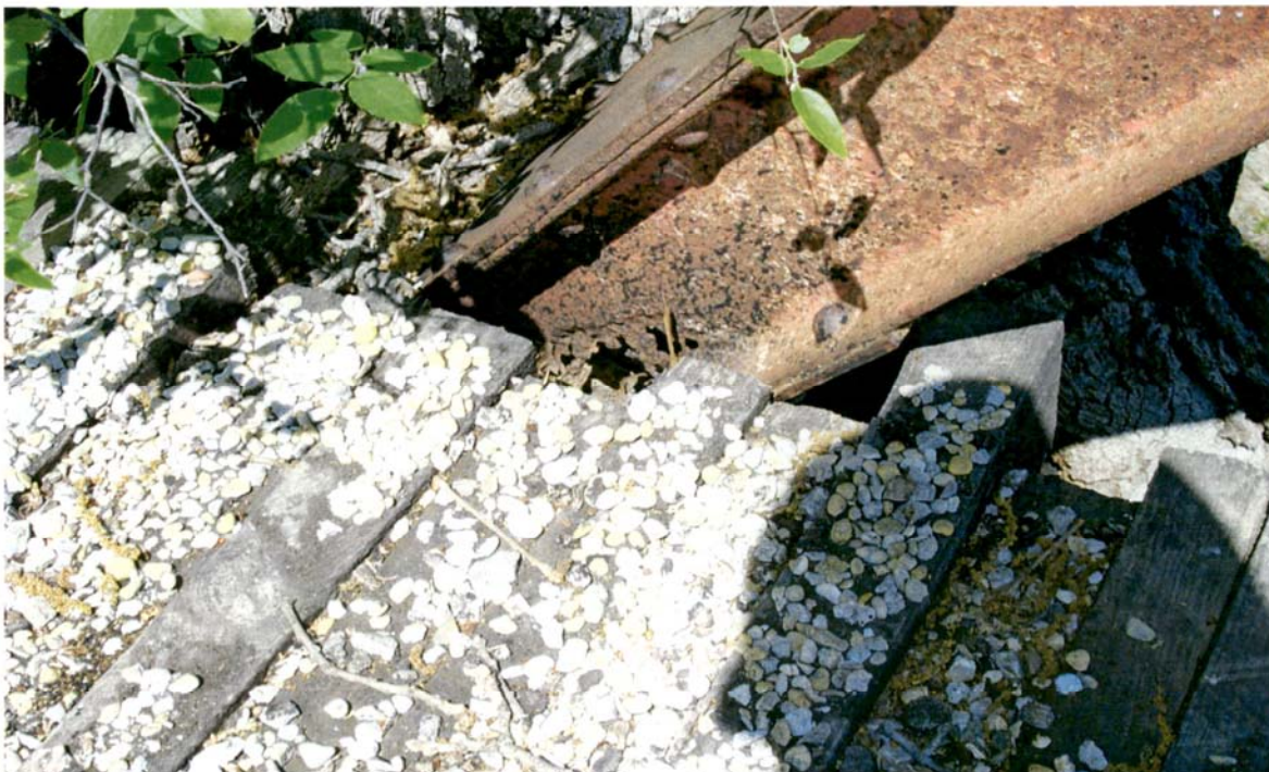
Rust Thru in South End Post of West Truss Rating: 4
