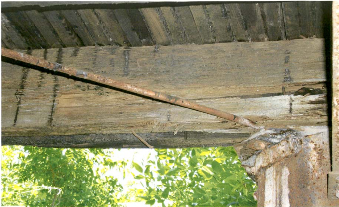
Severe Decay With Splits of Truss Timber Stringers Rating: 1
