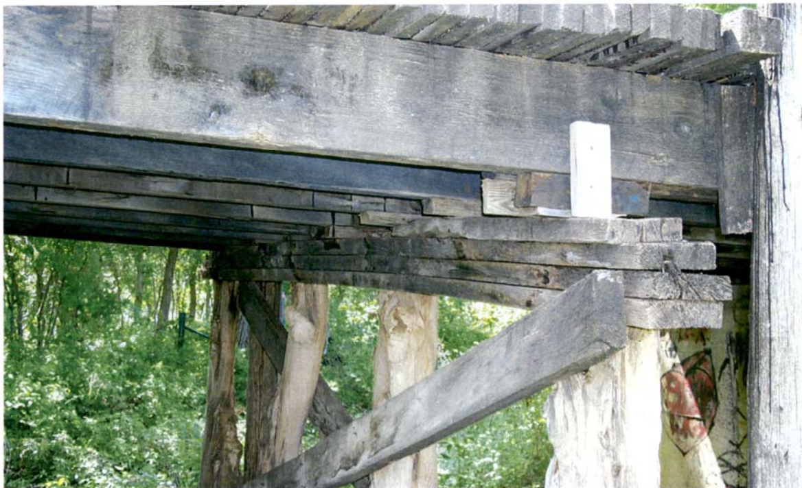
Differential Settlement Between East and West Ends of Bent #2 (From South) Rating: 1
